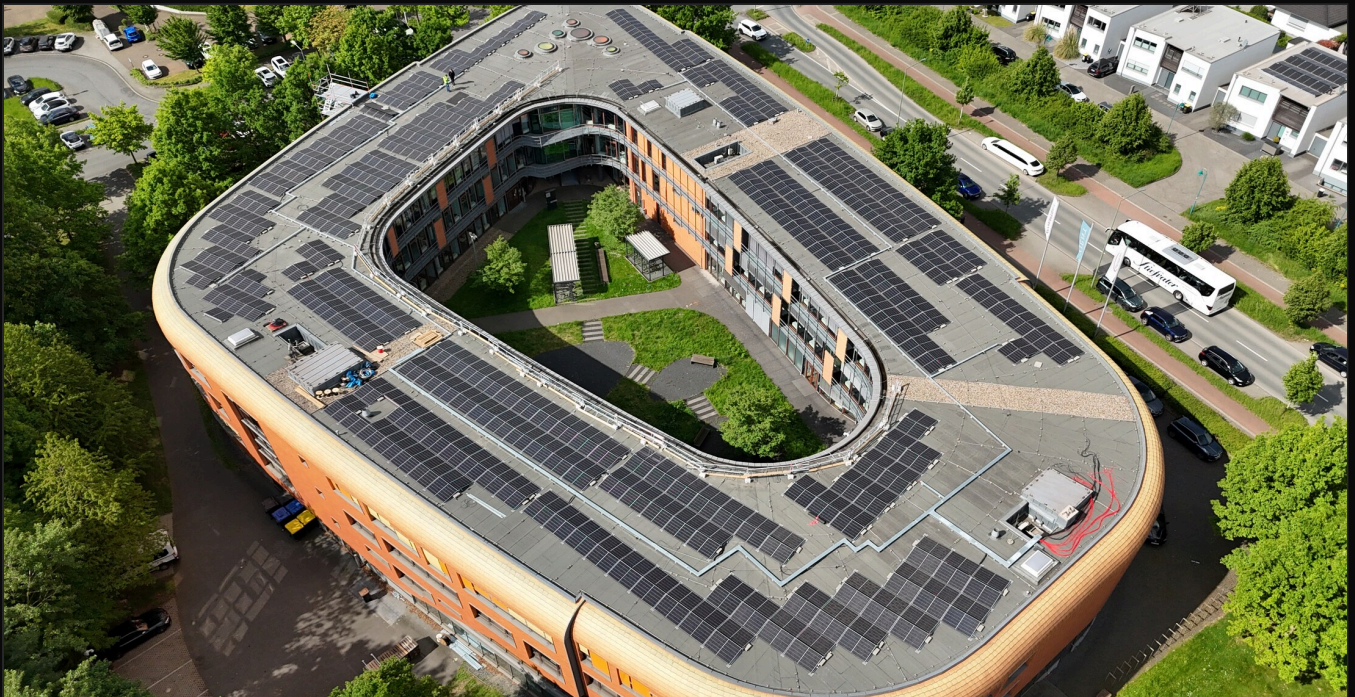
Solar roof & landscaped courtyard – the building from above.
